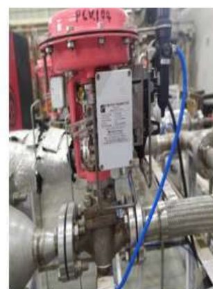
Figure A.4.26: Indigenously developed pressure control valve for helium service.
