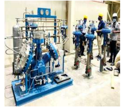
Figure A.4.14: Installation of EHCL components.
