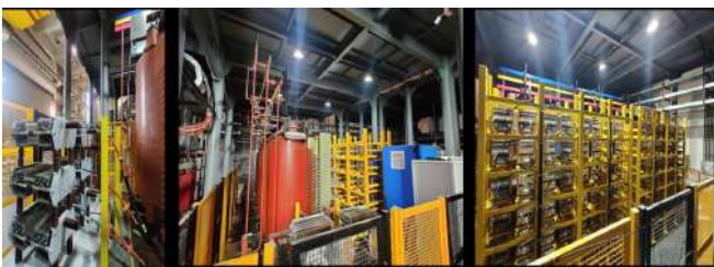
Figure B.1.22: Operations of the 55 kV, 6 MW MVHPS with the dummy load prior to its integration with the gyrotron
