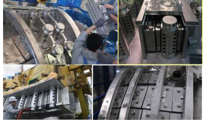
Figure B.1.5: In sequence : IWS lowered for assembly in VV sector, IWS assemble around flexible support housing between outer and inner shells of VV, inspection after assembly to ascertain needed clearance, VV segment view after assembly of IWS and ready for welding the outer shell.
