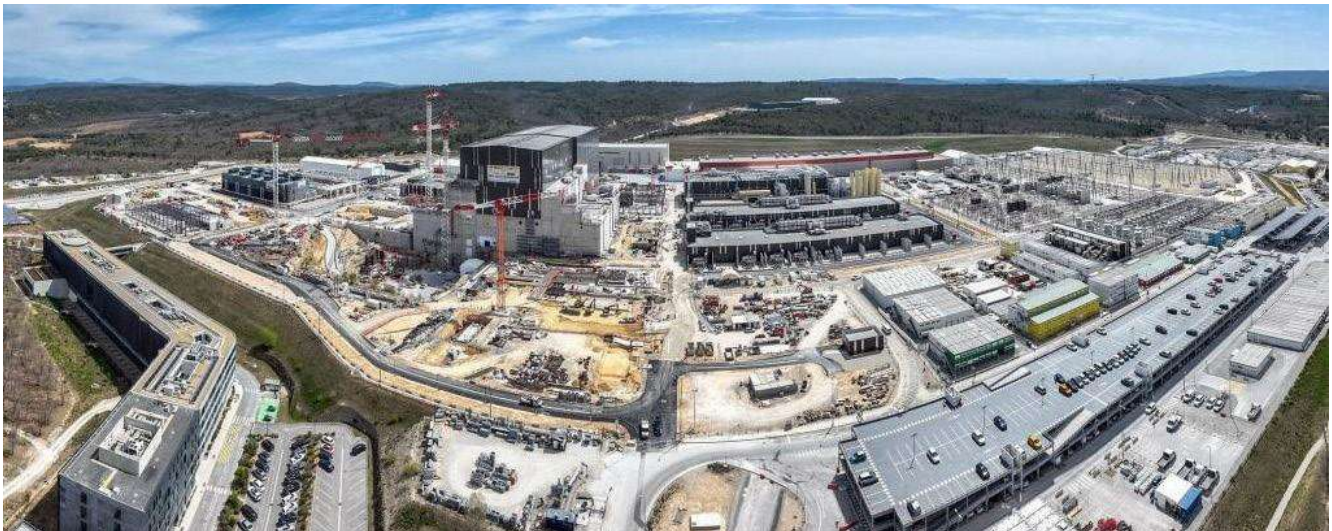
Figure B.1.1: Aerial view of the ITER site.
